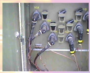
Hot Spot Temperature....159F Reference Temperature....98F Temperature Difference...61F Ambient Temperature....71F
