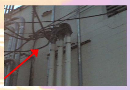
Hot Spot Temperature...301F Reference Temperature...77F Temperature Difference..224F Ambient Temp......45 F
