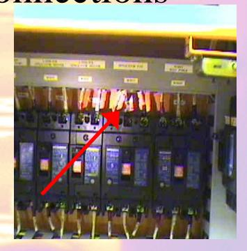
Hot Spot Temperature.....459F Reference Temperature.....101F Corrective Measures Required Temperature Difference....358F
